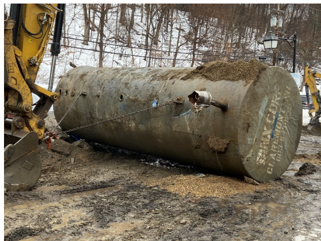
Service station tank removal
